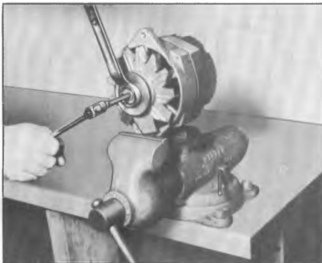
Fig. 10c—Pulley Removal
