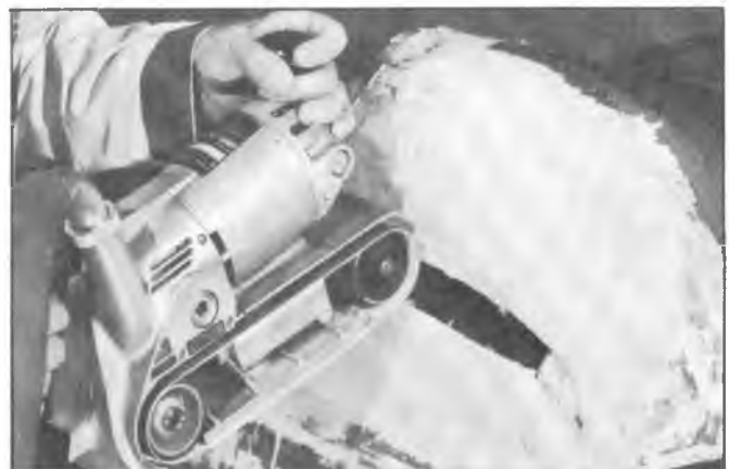
Fig. 54—Grinding "V" at Damaged Areas
